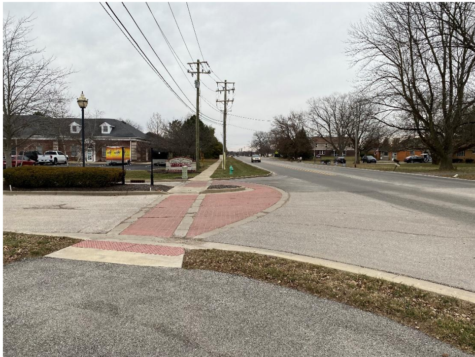
2) Existing access to CR 150 S / Oriole Way, facing east.
